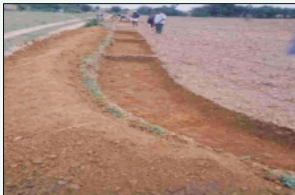
Trench-cum-bund in Tumkur cluster
