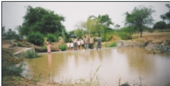
Check dam filled to brim during first rain in Mahabubnagar
