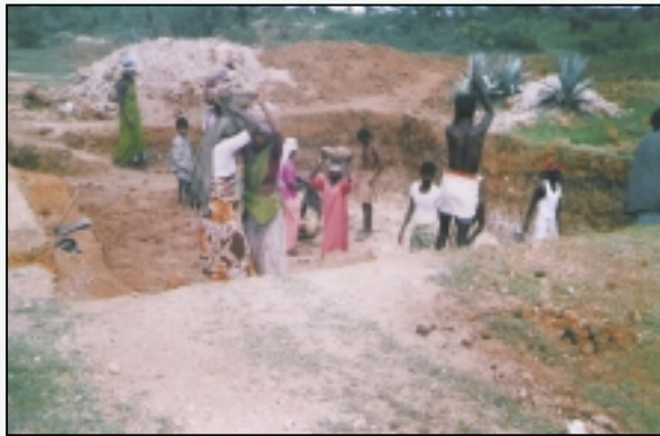
Digging of farm pond by villagers at Anantapur cluster
