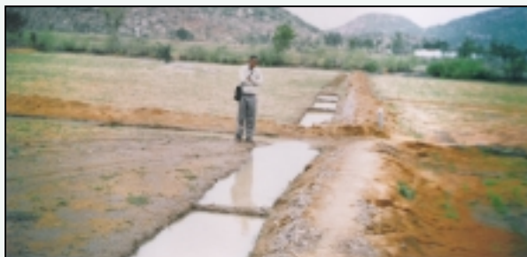
Trench cum bund for conservation of soil & water in Mahabubnagar
