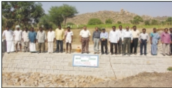
Check dam at Chowderpalli in Mahabubnagar
